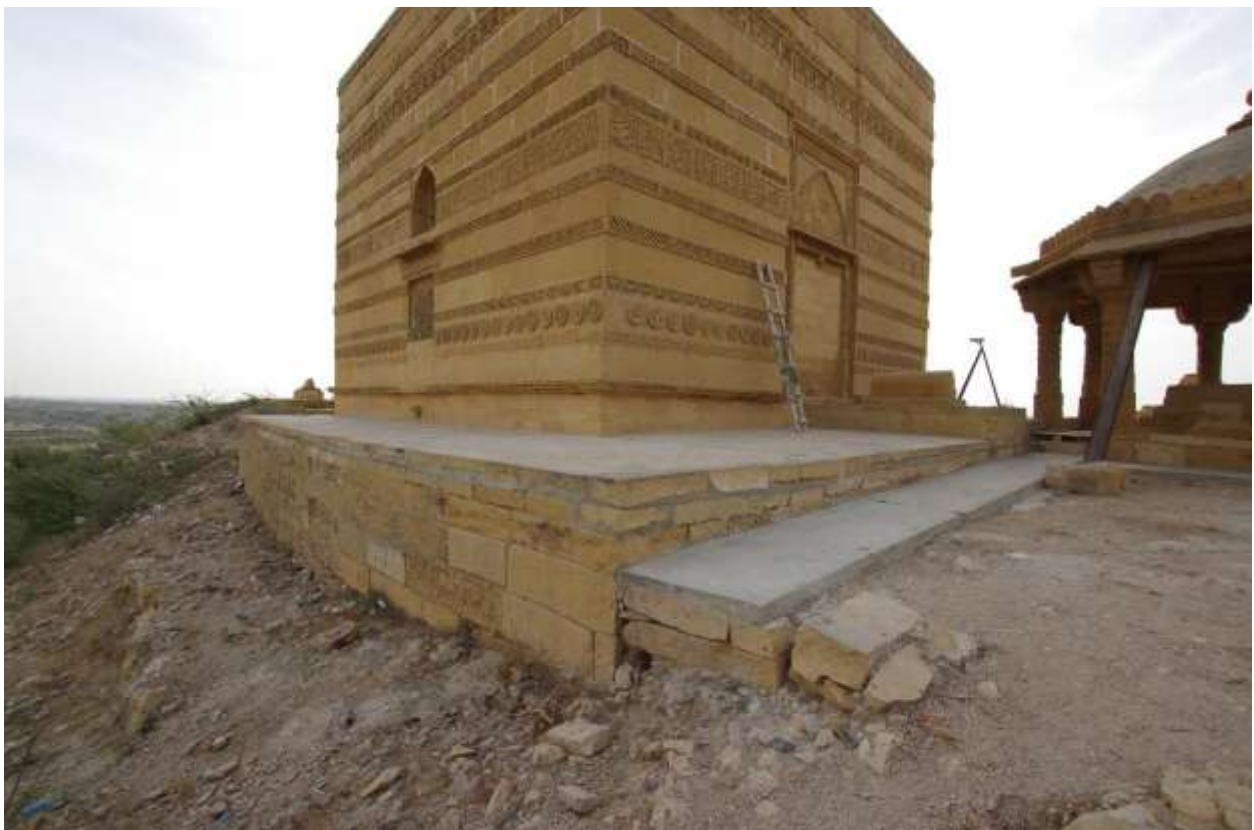
Image 14: North-east corner of Jam Nizam al Din with the encased retaining wall (built in 1994) and – below, right side, the newly added apron made of cement mortar for rainwater protection.
