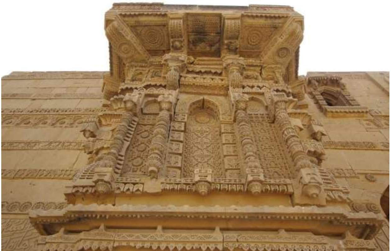
Image 24: Central risalit, looking upwards, with severe cracks below the protruding balcony structure and elements bulging outwards left of the symmetry axis.
