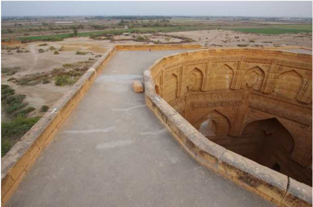
Image 35: Top level with cement flooring and the two added courses of stones (1956).
