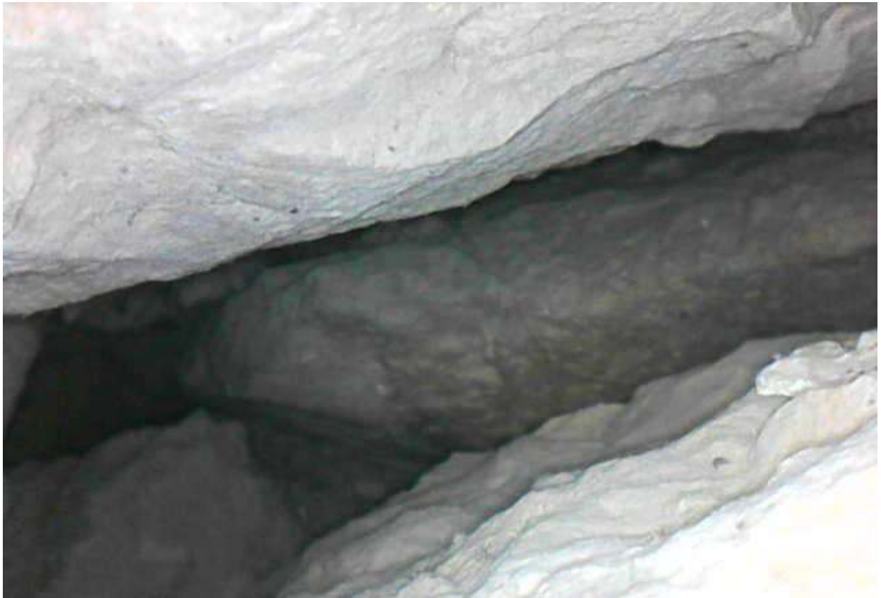
Image 37: Endoscopic view of a cavity next to the gateway at the northern wall, showing the inner layer of rubble stones.
