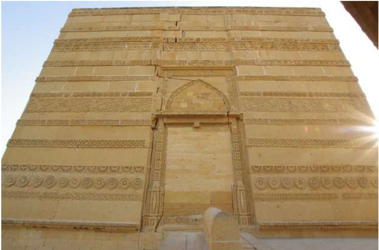
Image 11: North facade of Jam Nizam al Din, showing the sealed northern doorway and the series of cracks above.
