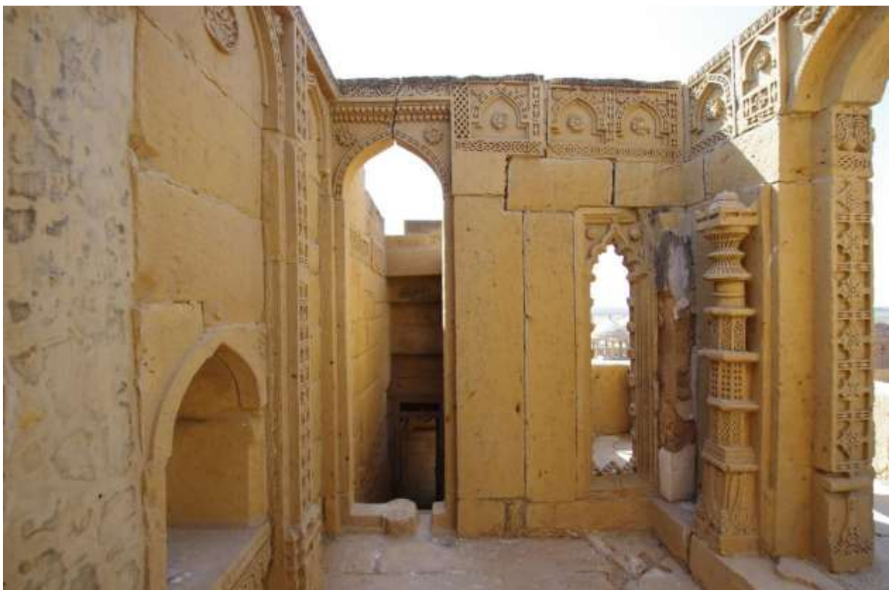
Image 30: Vestibule of the Darshan Jharoka, looking south, with the broken lintel above the doorway.
