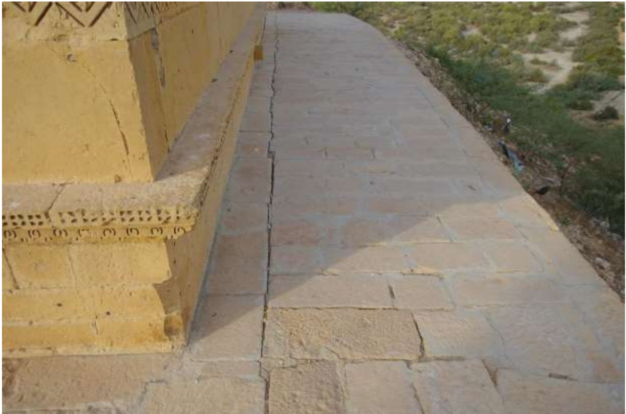
Image 13: Encasement of the added retaining wall (1994), showing a horizontal gap with increasing width from south to north. Note that the waterspout that drains the central space dewateres directly into the crack between the foundation wall and the newly built retaining wall, which is encased in the plinth (built in 1994). The water is trapped in the gap in between and is funnelled directly to the moisture-sensitive clayish layer below the foundation walls.
