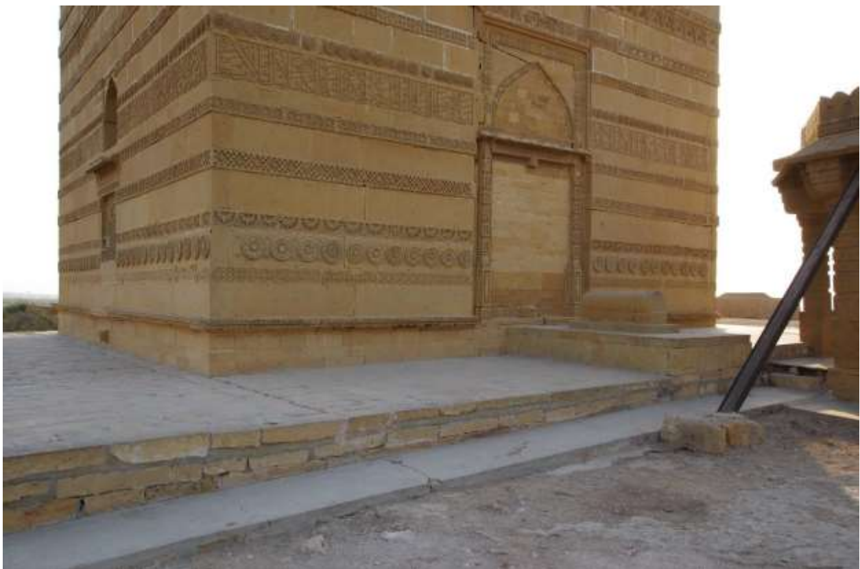
Image 10: North-eastern corner of the building with the masonry encased retaining wall installed in 1994 and (in the foreground) the concrete apron installed in 1996.
