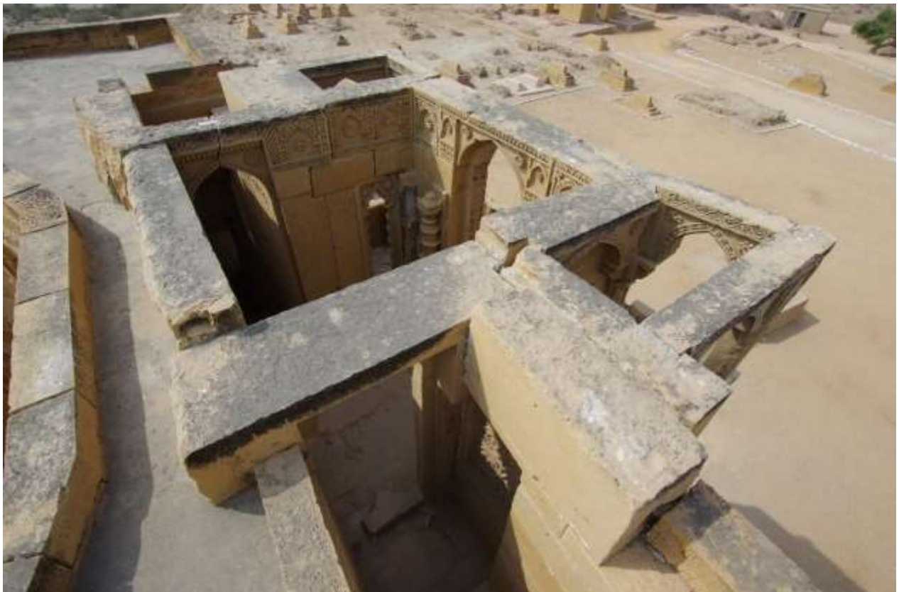
Image 34: Top view of the balcony structure, showing the severe dislodgements and misalignments.
