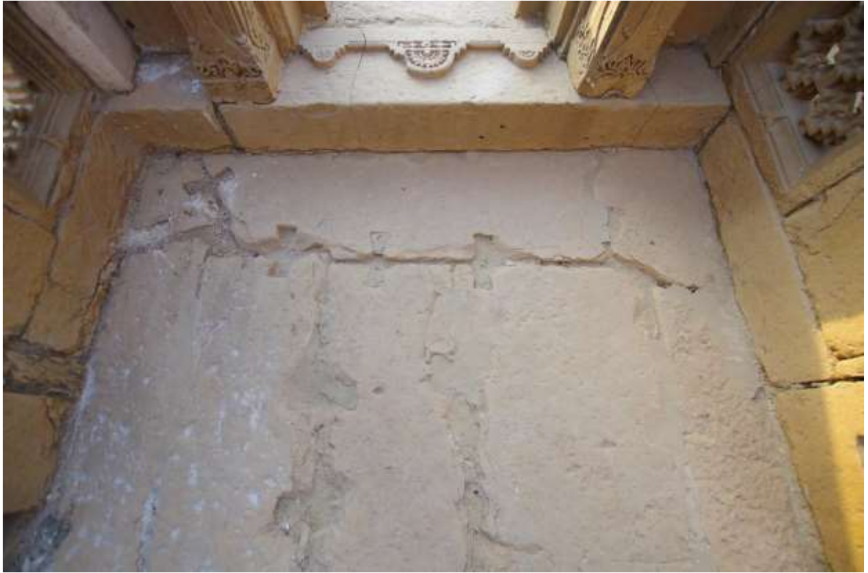
Image 31: Vestibule of the Darshan Jharoka, stone planks with missing iron clamps.
