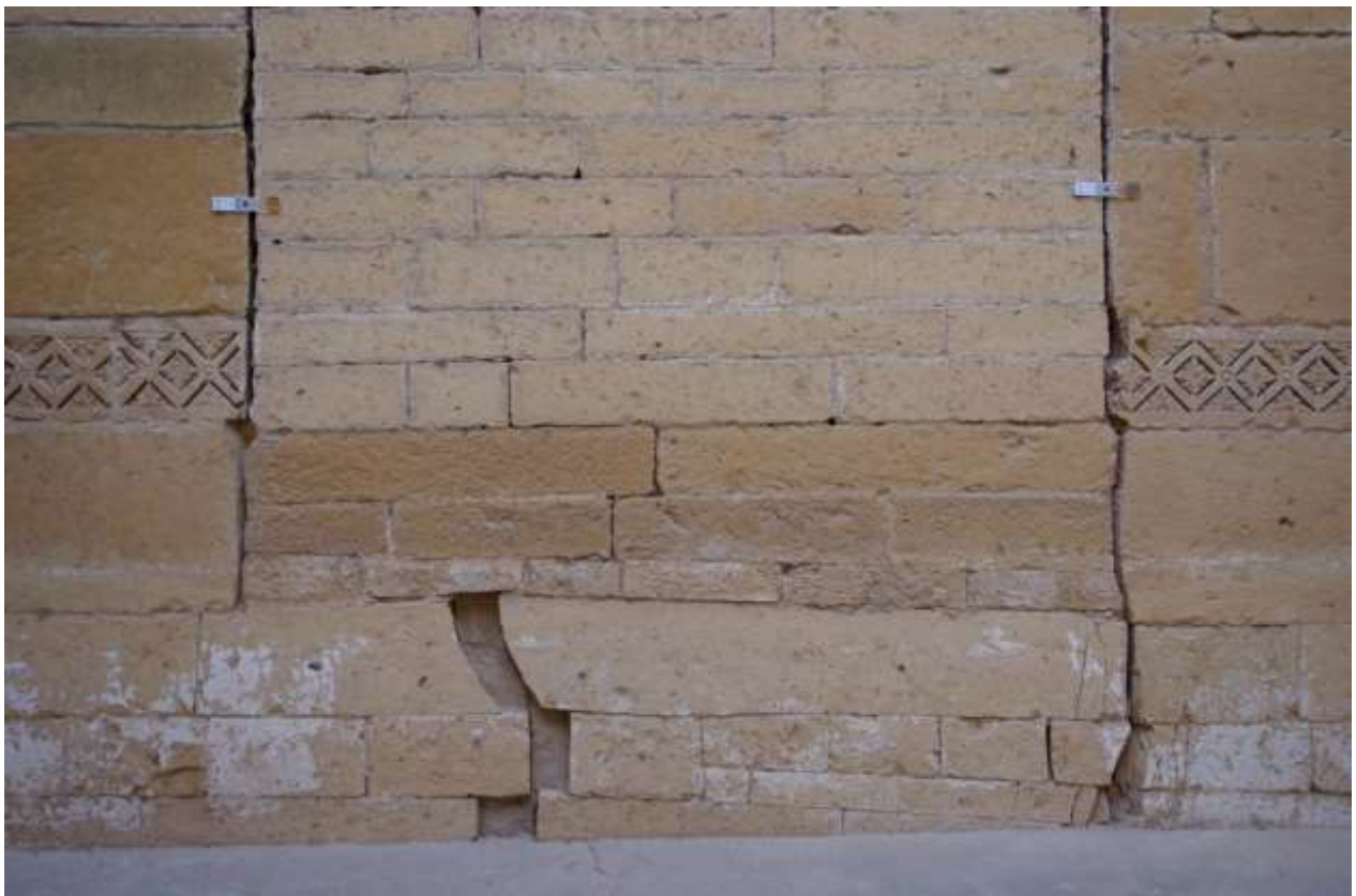
Image 18: Sealed northern doorway with installed crack-meters. The lower (previously sealed!) crack through the lowest three courses shows very clearly that the foundations of the monument are not only subject to vertical settlement but also to horizontal sliding.
