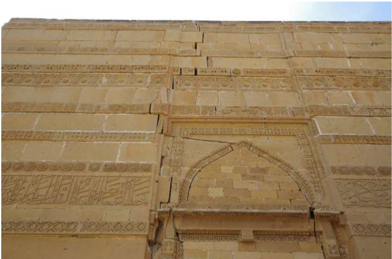
Image 12: Upper part of north façade with opening gaps between the stone elements (some former infill patches caved outwards and are missing, the maximum opening since 1994 measures approx. 18mm.)
