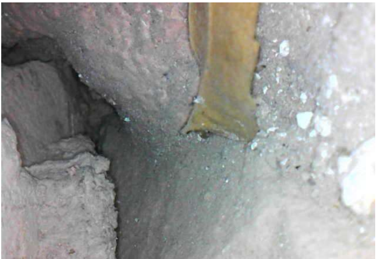
Image 38: Endoscopic view of crack between the detached central pilaster and the main structure. It shows a patched crack within the mihrab niche (taken from the opposite site).
