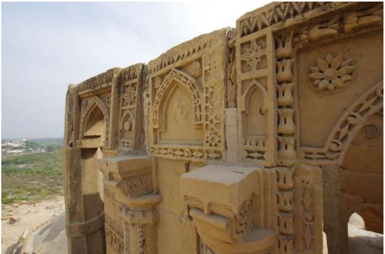
Image 32: Upper entablature of balcony structure, looking north. The disruption and perturbation of the structural elements is clearly visible, with wide (partly repointed) gaps, dislodgements and misalignments and lost original elements (e.g. post on the left hand side).
