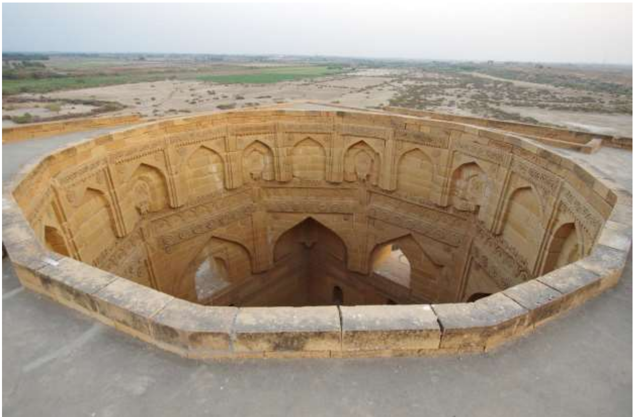
Image 36: Top level with cement flooring and the two added courses of stones (probably carried out in 1956 by the department of public works).
