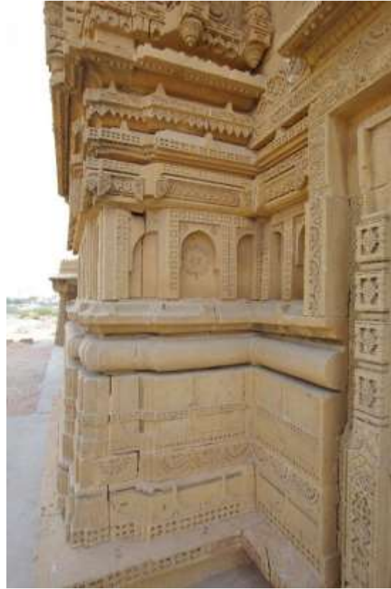
Images 25 a/b: Lower part of central risalit from north / south – with a continuous vertical gap on the north side.
